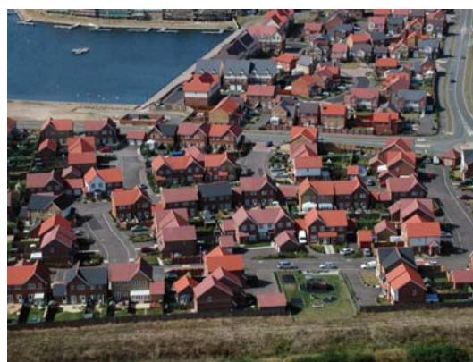
Housing Development in Sovereign Harbour
