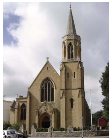
Our Lady of Ransom Catholic Church - Grade II Listed Building
